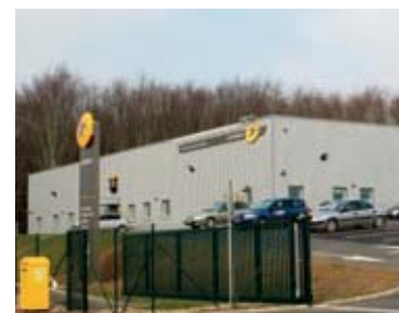
> The Mail preparation and delivery hub in Saint-Lô was built in line with the "Bâtiment Basse Consommation" (low-energy building) label.
